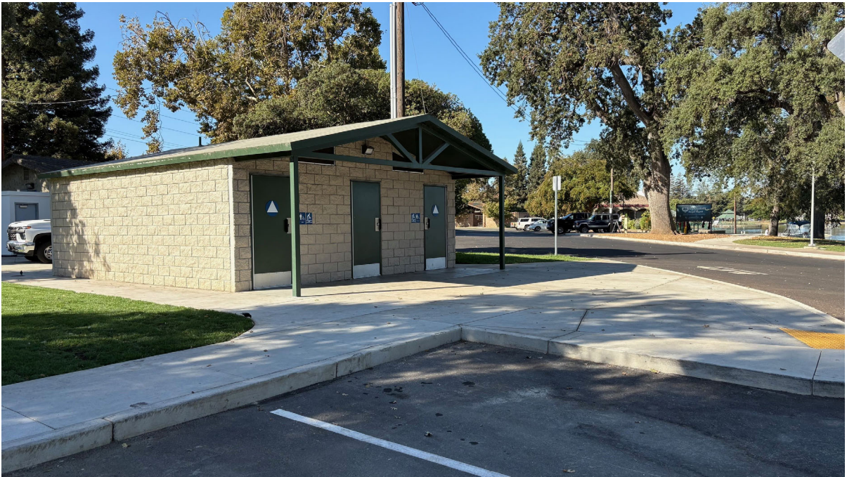
South Restroom Building
