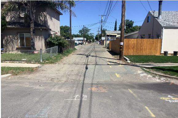
West Alley Approach Before
