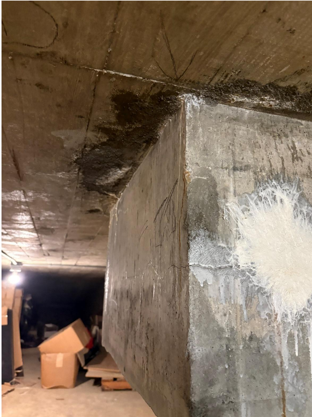
Photo 5 – Concrete drain box
