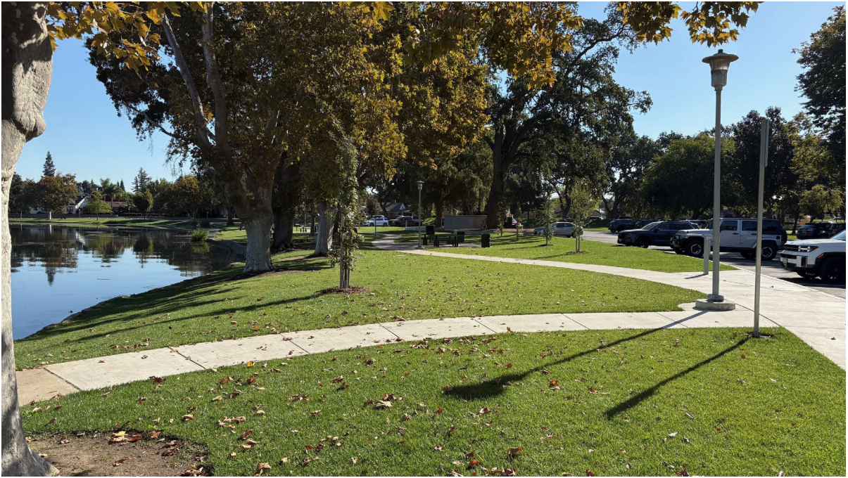
Southern Parking Lot Walkway Improvements
