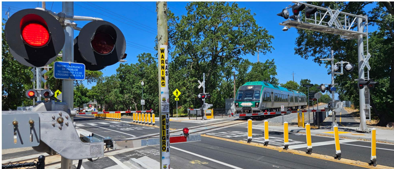
Figure 2. Town of Windsor Mitchell Drive 100' Channelization Example
