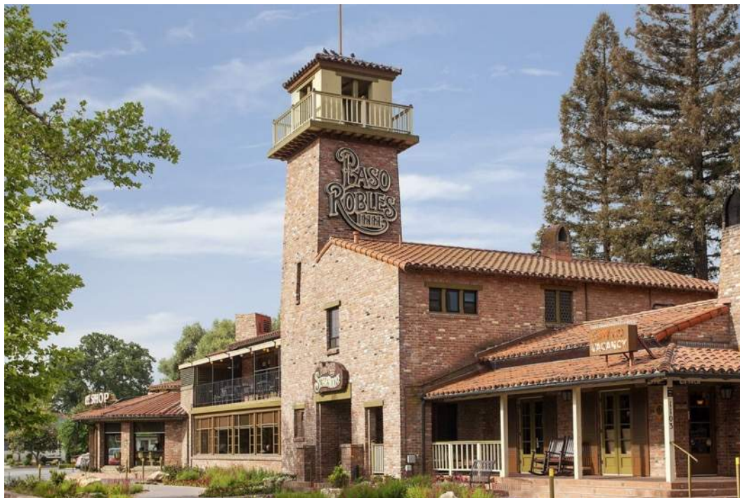
Figure 6: Rebuilt Historic Paso Robles Inn
